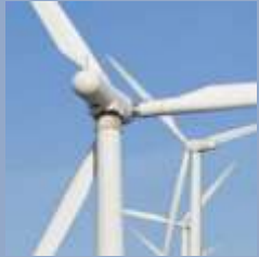
Use of renewable energy.
